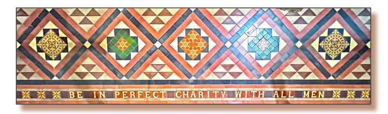
A restoration of the installation in 2023 required work on around 150 tiles, including their removal, repair or replacement, reinstatement, consolidation, and grouting, followed by cleaning, sealing and polishing. This work was made possible by a legacy left to us by our late friend Jim Storr – a loyal and longstanding member of the congregation of Holy Trinity Church. We are confident that he would have been supportive of this project, and delighted with its outcome.
